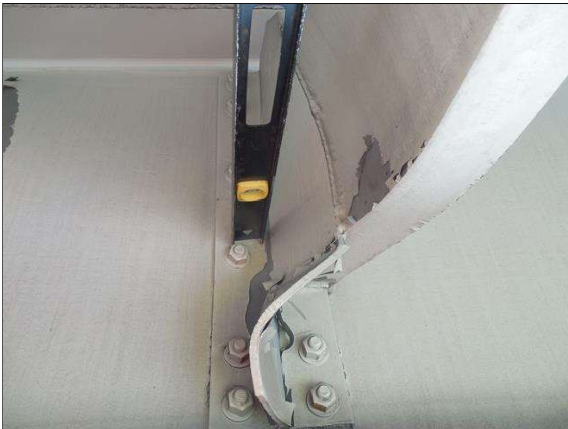
SPAN 4 BAY 4: BOTTOM HALF OF DIAPHRAGM #2 BENT TO THE WEST APROX. 8" AT BEAM 5 CONNECTION.
