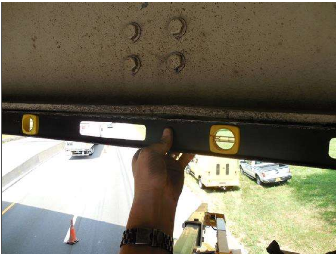
Span 4 Beam 3: 4"L SECTION ALONG SOUTH EDGE OF BOTTOM FLANGE AND COVER PLATE BENT UP 3/16", LOCATED 19'-6" FROM BENT 4 BEARING
