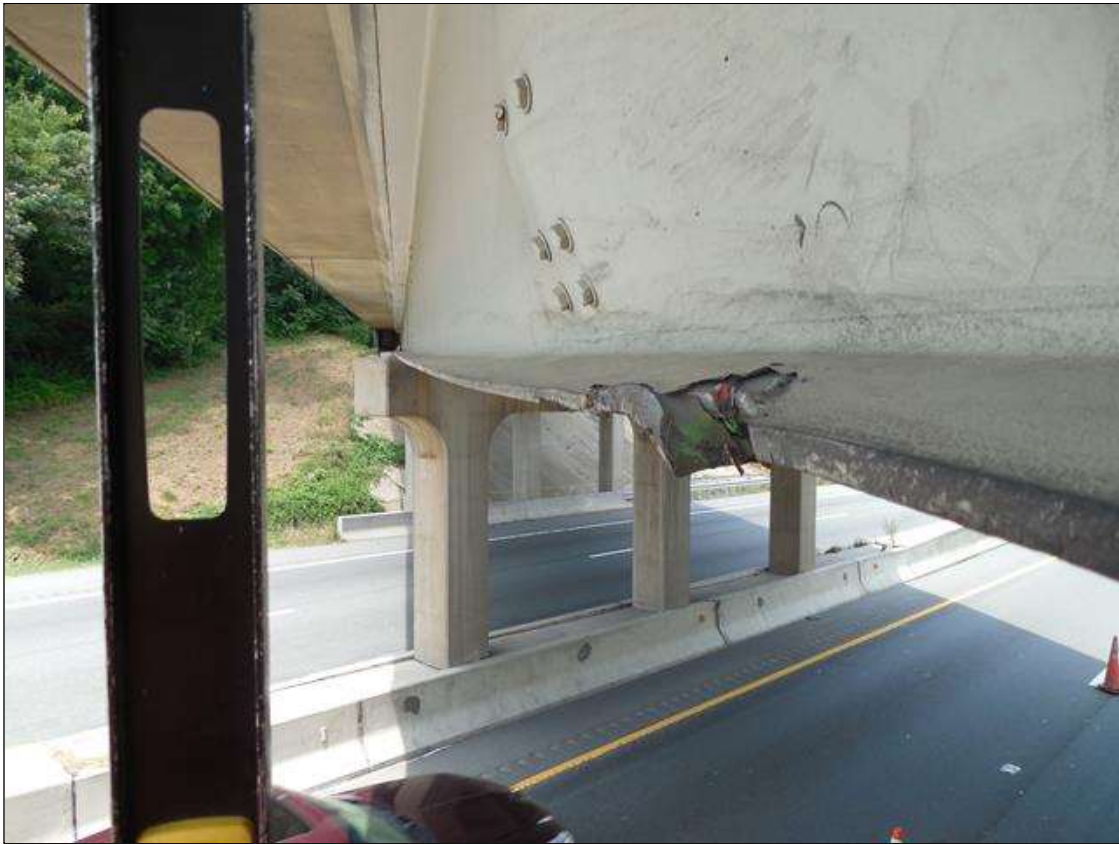
Span 4 Beam 5: INITIAL POINT OF IMPACT (POI) AT 17'-6" FROM BENT 4 BEARING. BEAM OUT OF PLUMB 9" TO THE NORTH AT POI - TOTAL OF 30LF OF BEAM DEFLECTED FROM INT. DIAPHRAGM #1 IN BAY 4 TO BENT 4 BEARING.
