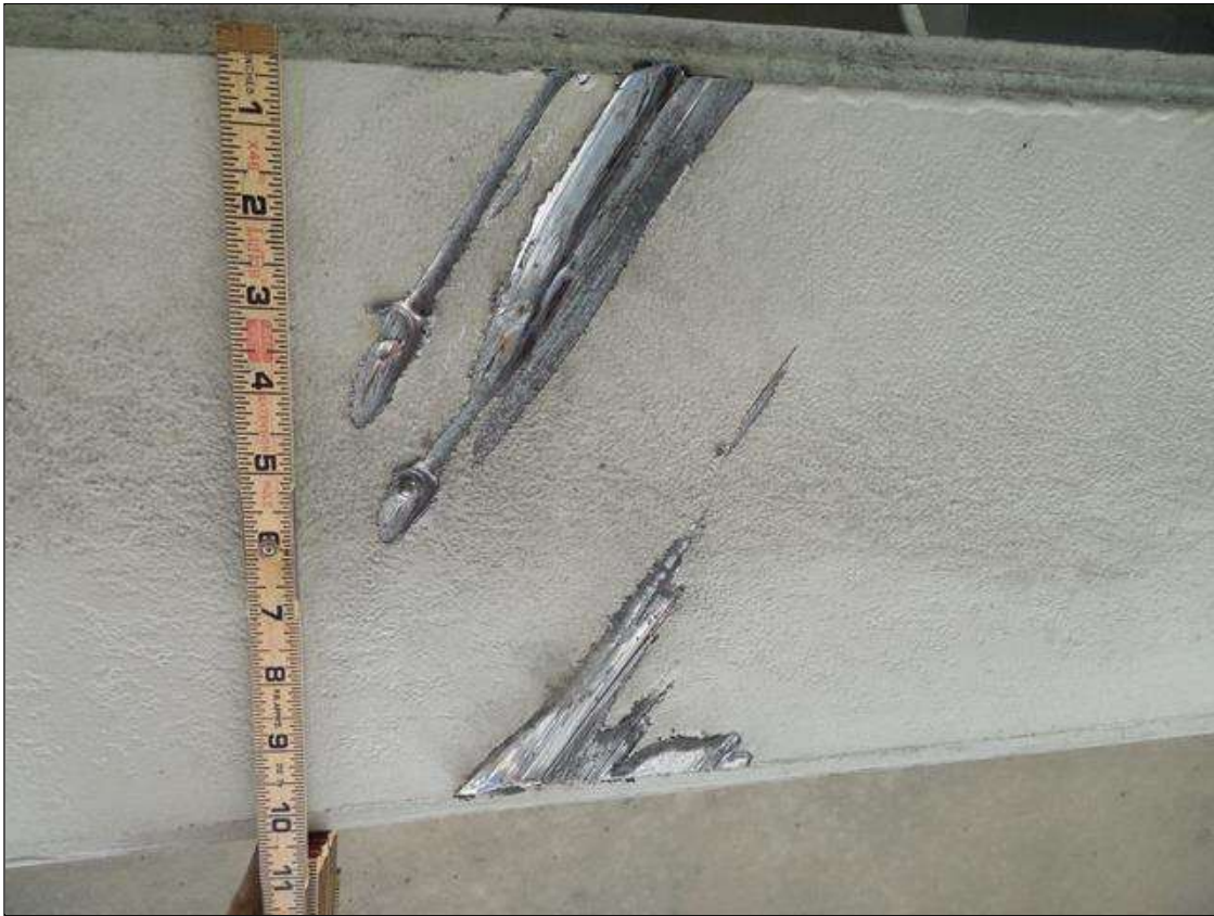
Span 4 Beam 4: (2) 3"L x 6"W AREAS OF 1/8"D SCRAPES ON BOTTOM COVER PLATE, LOCATED 19'-6" FROM BENT 4 BEARING
