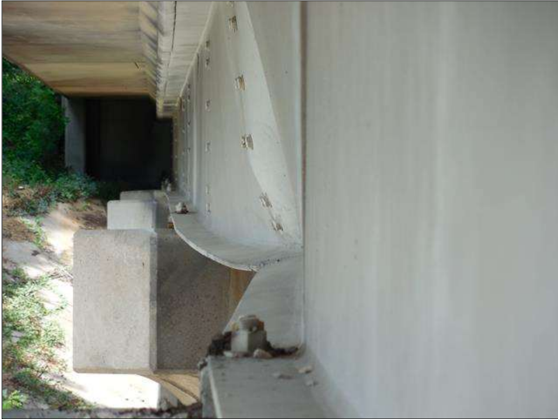
Span 4 Beam 5: LOOKING WEST ALONG SOUTH SIDE - INITIAL POINT OF IMPACT (POI) AT 17'-6" FROM BENT 4 BEARING. BEAM OUT OF PLUMB 9" TO THE NORTH AT POI - TOTAL OF ~30LF OF BEAM DEFLECTED FROM DIAPHRAGM #1 IN BAY 4 TO BENT 4 BEARING.
