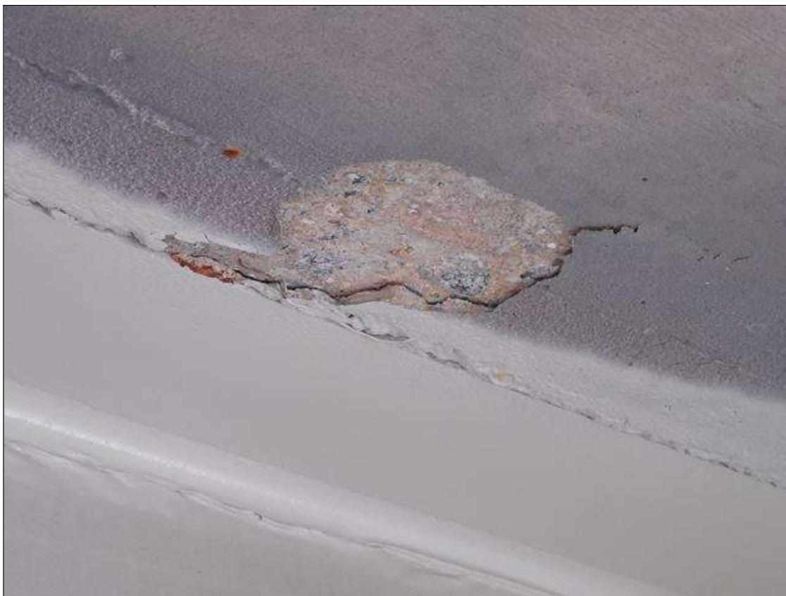
Span 4 Deck: 1/4"D x 6" DIAMETER SPALL IN BOTTOM OF DECK AT TOP FLANGE OF BEAM 5 IN BAY 4 LOCATED 20' FROM BENT 4
