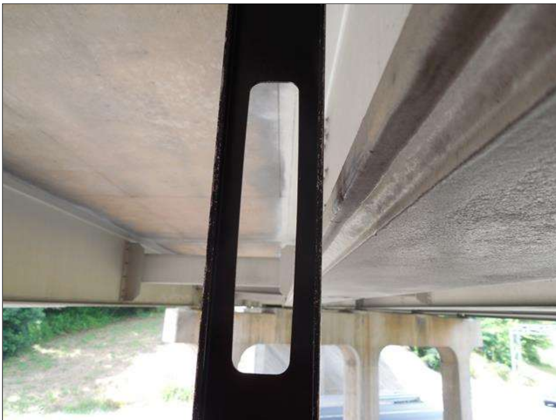
Span 4 Beam 4: 10LF OF BEAM OUT OF PLUMB 1/4" TO THE NORTH - CENTER POINT AT DIAPHRAGM #2 CONNECTION
