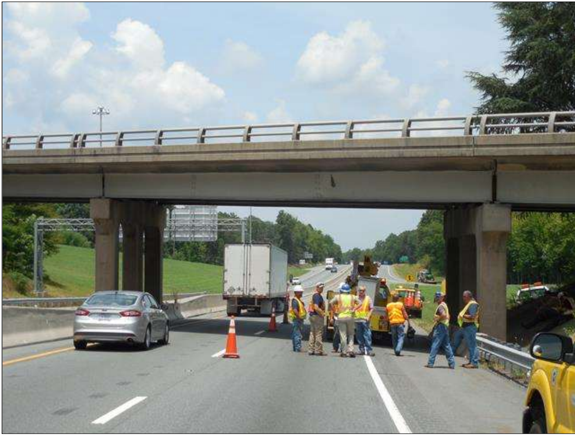
LOOKING NORTH THROUGH SPAN 4
