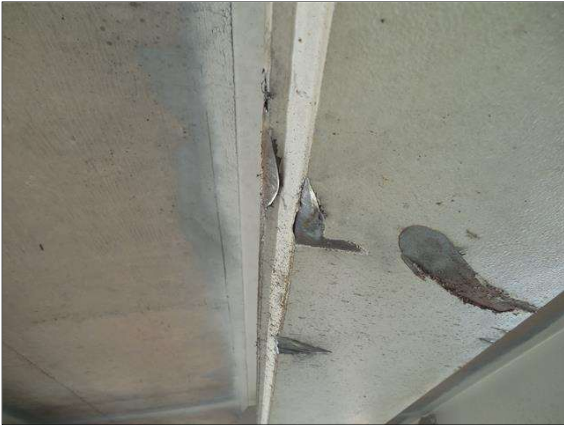
Span 4 Beam 3: (2) 2"L x 1/2"W x 3/16" INDENTIONS IN SOUTH EDGE OF BOTTOM COVER PLATE AND BOTTOM FLANGE LOCATED 19' FROM BENT 4
