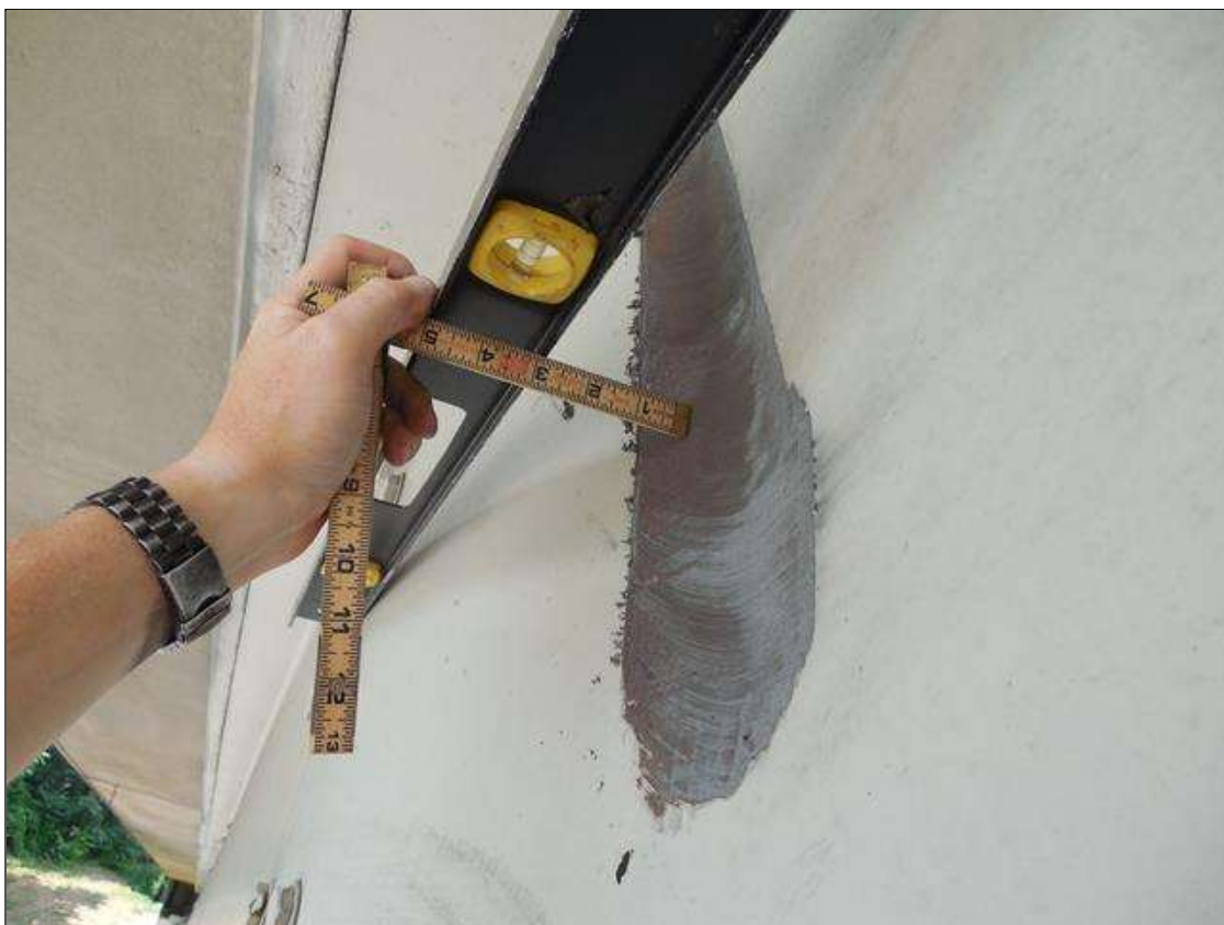
SPAN 4 BEAM 5: 17"H x 36"W x 3"D DEFORMATION IN WEB AT POI, BEGINNING 3" FROM TOP FLANGE
