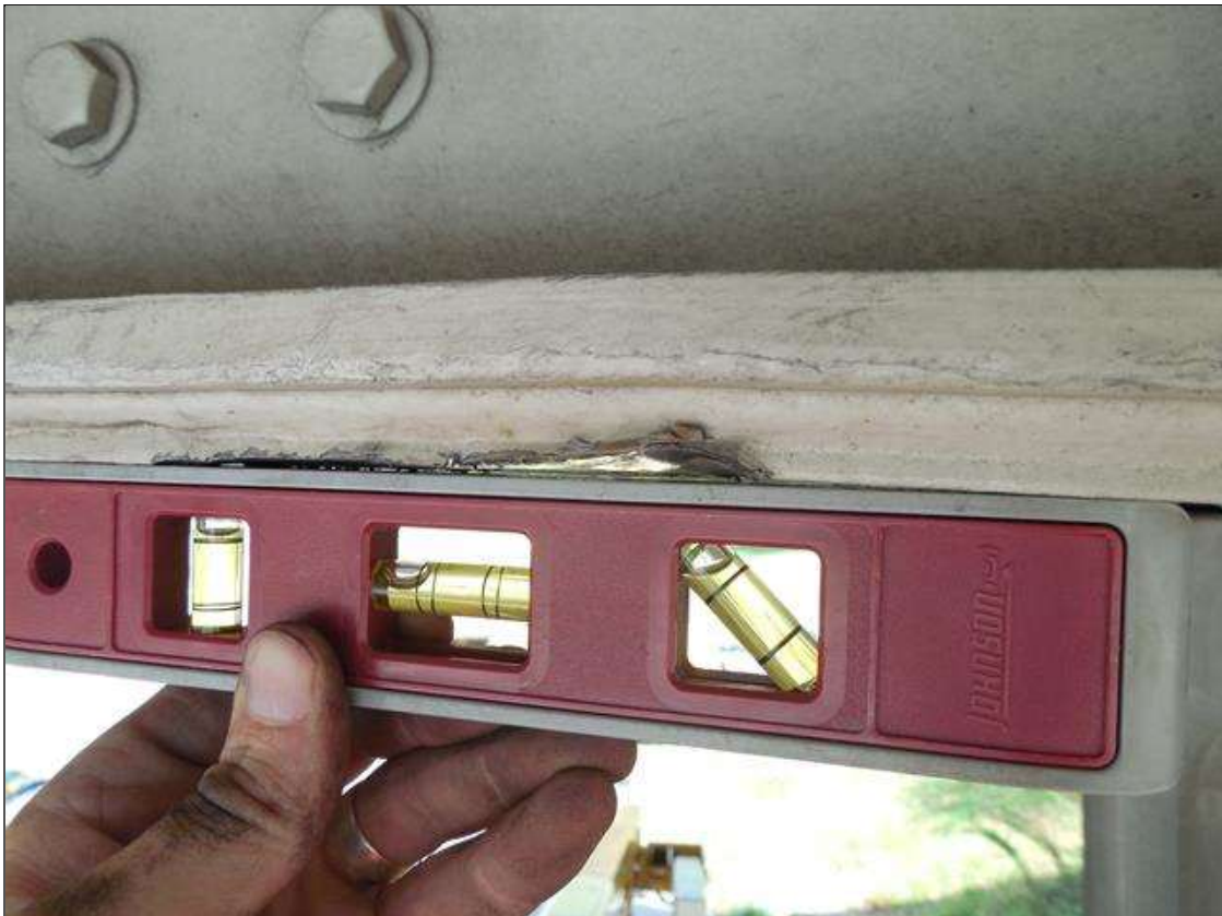
Span 4 Beam 4 : ALT. VIEW - (2) 3"L x 6"W AREAS OF 1/8"D SCRAPES ON BOTTOM COVER PLATE, LOCATED 19'-6" FROM BENT 4 BEARING
