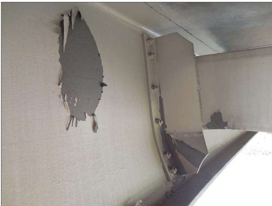
SPAN 4 BEAM 5: OVERVIEW OF NORTH SIDE OF DAMAGE TO BEAM WEB AND DIAPHRAGM #2 AT POI
