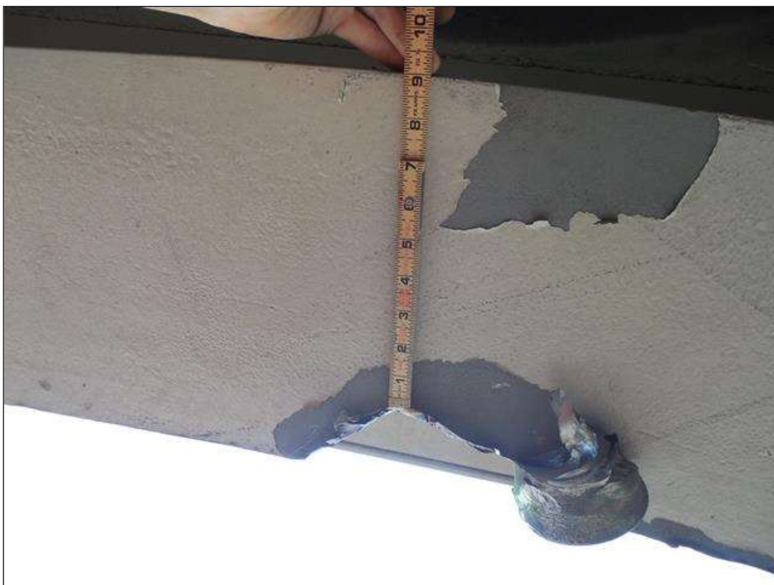
SPAN 4 BEAM 5: BOTTOM VIEW OF 7"L x 2-3/4"W TEAR IN SOUTH HALF OF BOTTOM FLANGE AT POI - 9" OF BOTTOM FLANGE REMAINING.
