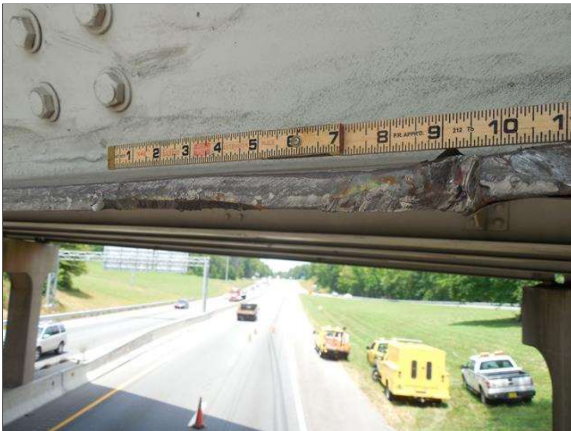
SPAN 4 BEAM 5: OUTSIDE EDGE OF BOTTOM FLANGE SCRAPED AND GOUGED UP TO 1/4"D ACROSS 11" AREA ADJACENT TO POI
