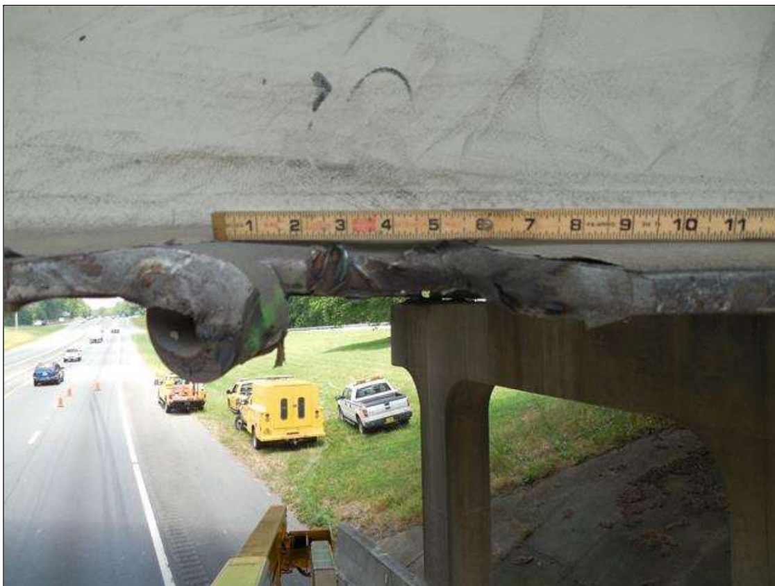
SPAN 4 BEAM 5: 7"L x 2-3/4"W TEAR IN SOUTH HALF OF BOTTOM FLANGE AT POI.
