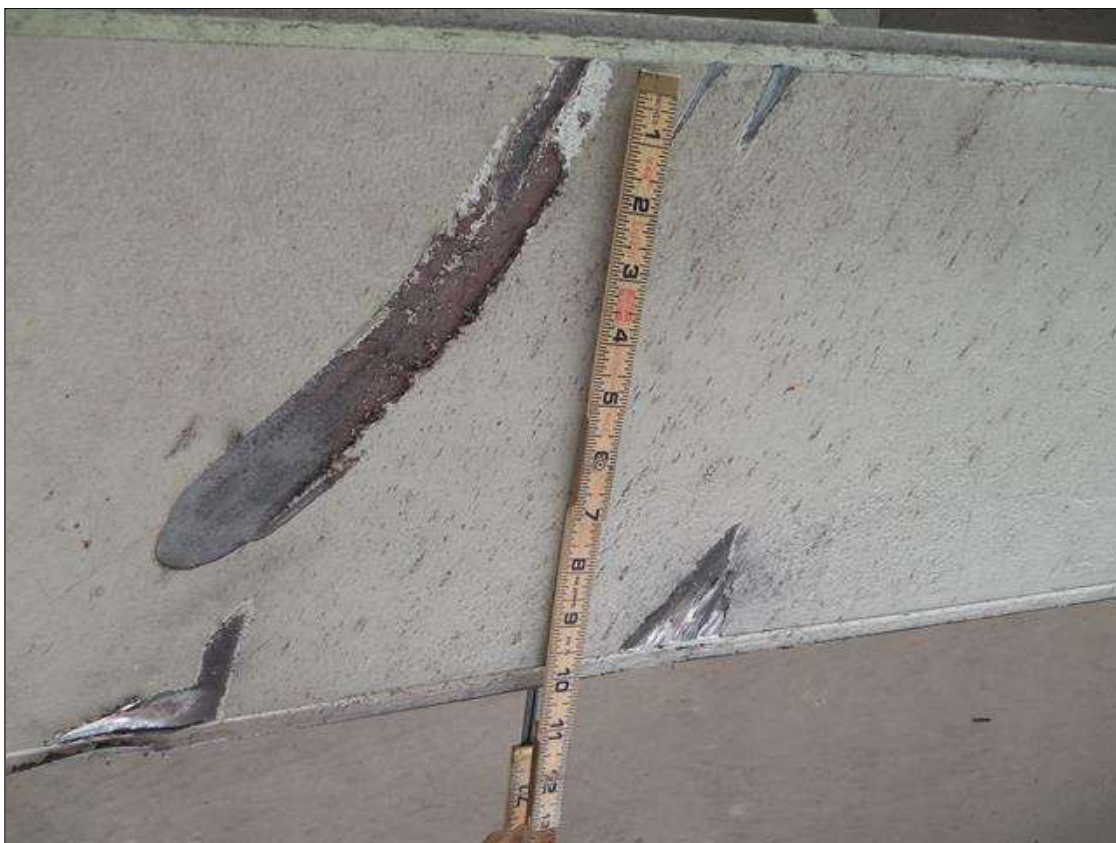
Span 4 Beam 3: 9"L x 2"W SCRAPE ON BOTTOM COVER PLATE APPROX. 1/32"D, LOCATED 19' FROM BENT 4 BEARING
