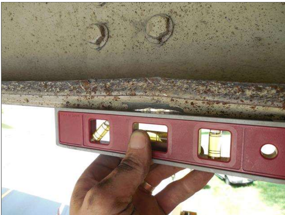
Span 4 Beam 3: 2"L x 2"W x 1/8"D GOUGE IN SOUTH EDGE OF COVER PLATE, LOCATED 19'-6" FROM BENT 4
