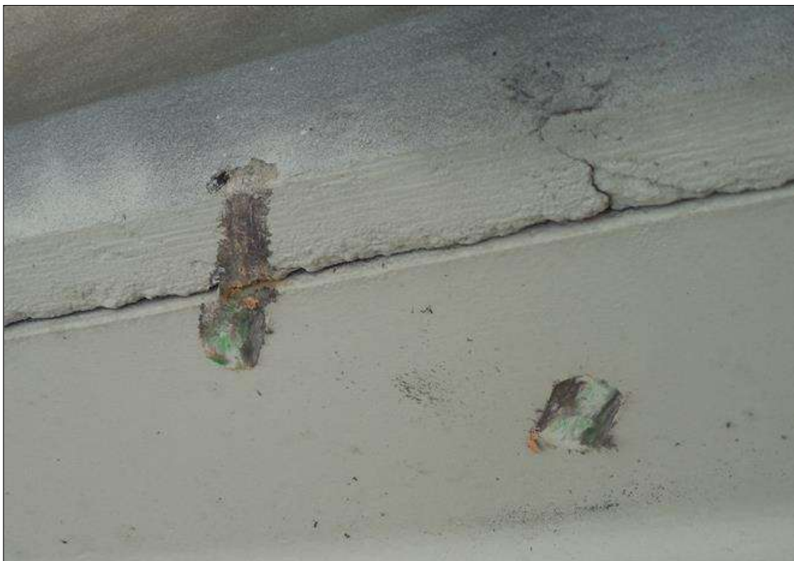
SPAN 4 BEAM 5: (2) 1" DIAMETER SCRAPES IN TOP FLANGE AT POI
