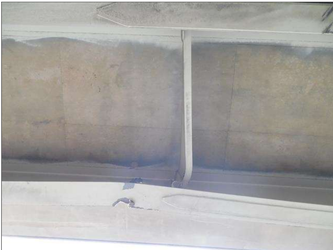
SPAN 4 BAY 4: LOOKING UP AT POI - BEAM 5, DIAPHRAGM #2, BEAM 4 SHOWN
