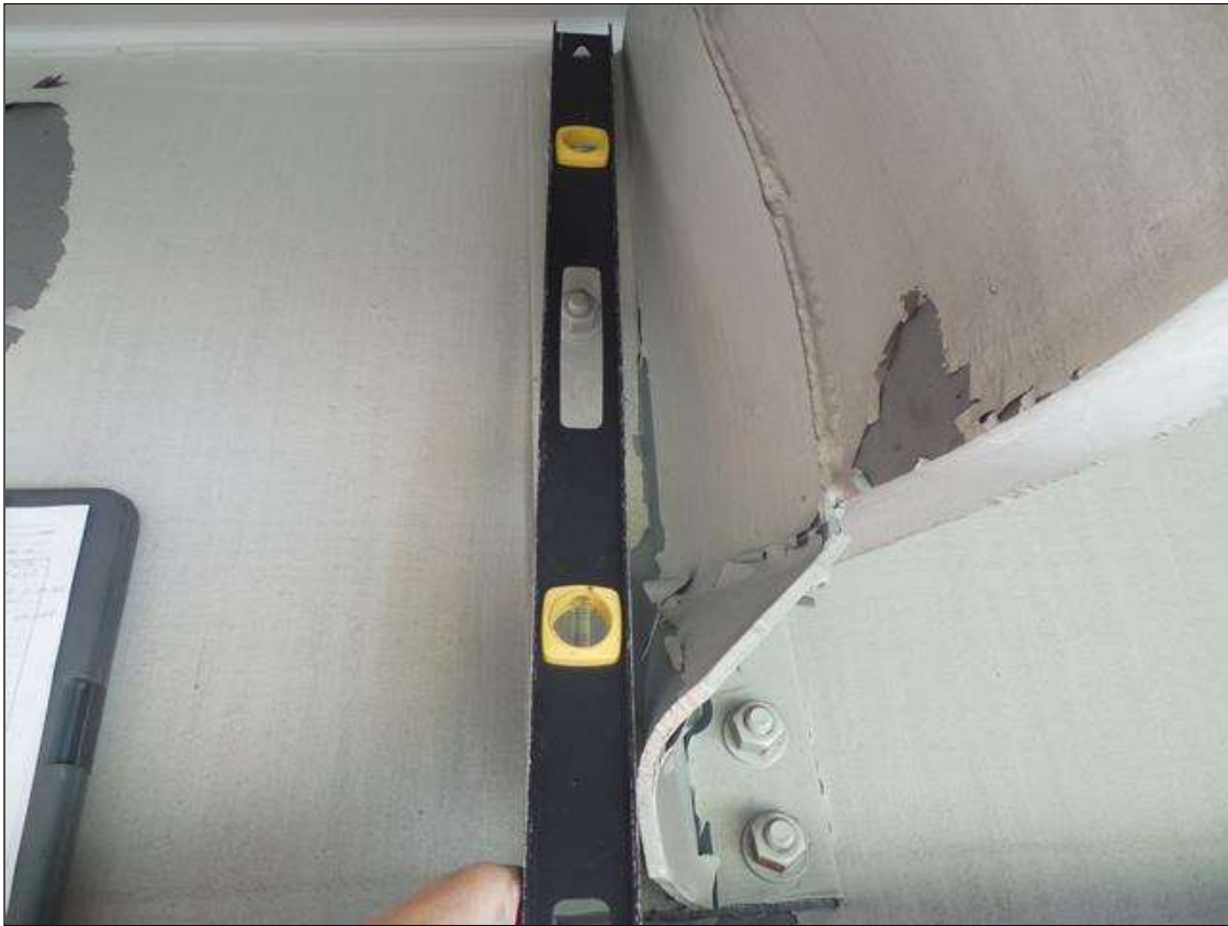
SPAN 4 BAY 4: DAMAGE TO ENTIRE LENGTH OF DIAPHRAGM #2 BEAM 5 CONNECTION BRACKET - MAX DEFLECTION OF 6" TO THE WEST.
