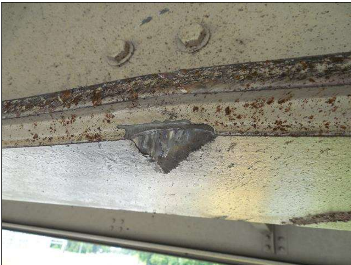
Span 4 Beam 3: ALT. VIEW - 2"L x 2"W x 1/8"D GOUGE IN SOUTH EDGE OF COVER PLATE, LOCATED 19'-6" FROM BENT 4
