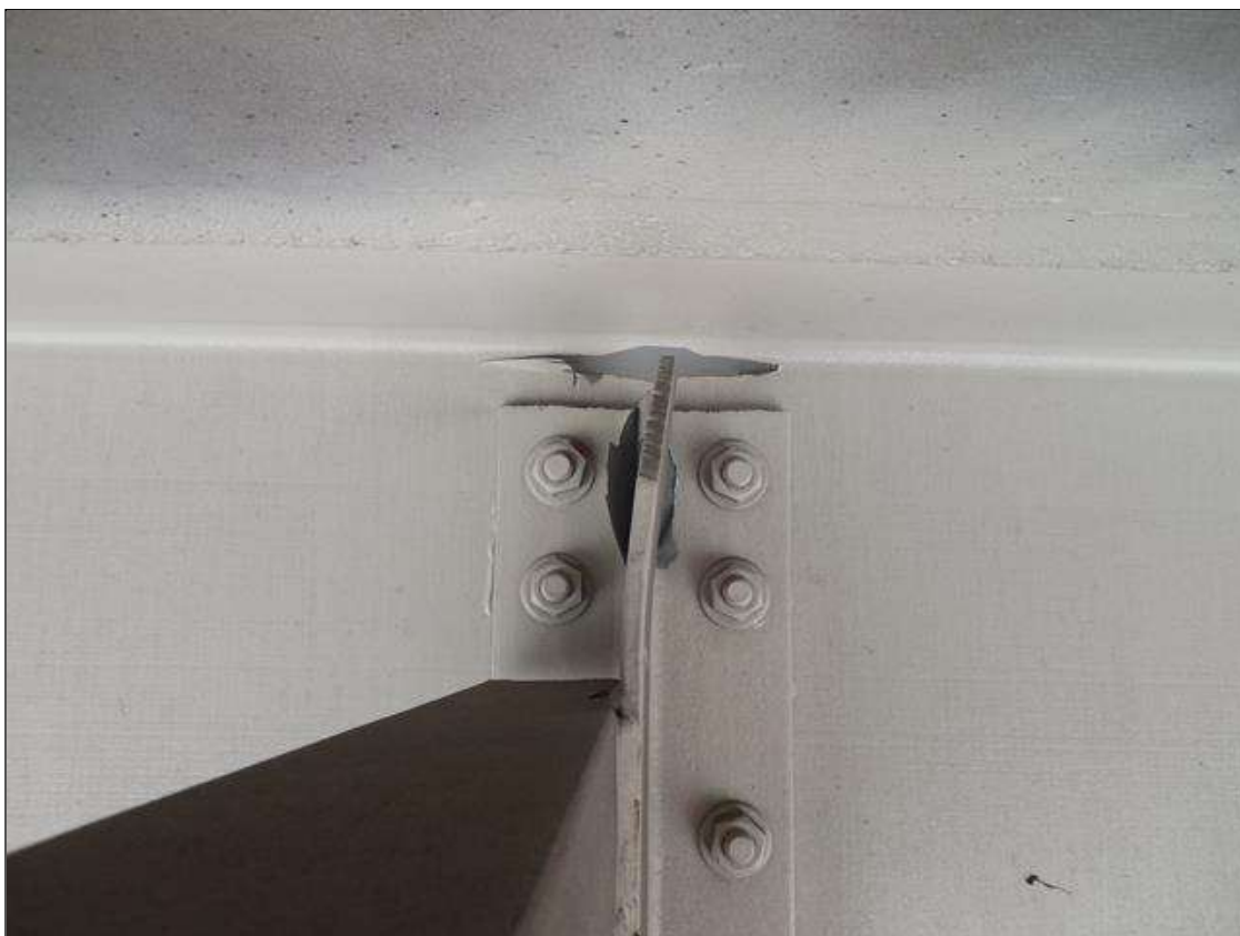
SPAN 4 BAY 4: TOP 4" OF DIAPHRAGM #2 CONNECTION TO BEAM 4 BENT 2" TO THE EAST
