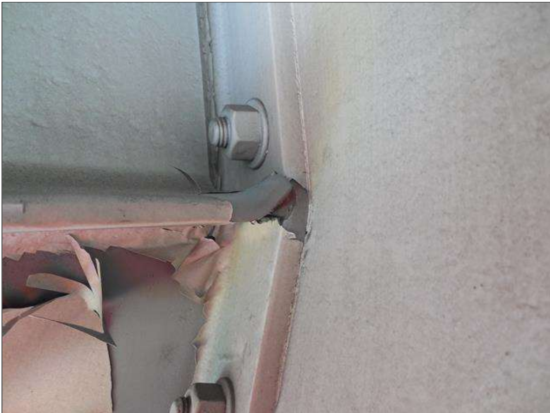
SPAN 4 BAY 4: 2"L x 1/2"H x 1/8"D INDENTION IN DIAPHRAGM #2 BEAM 5 CONNECTION BRACKET DUE TO CONTACT WITH DIAPHRAGM BOTTOM FLANGE
