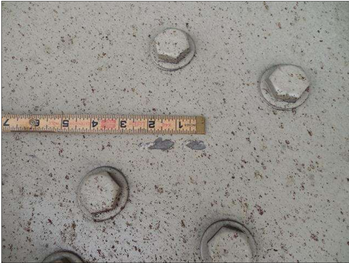
Span 4 Beam 3: APPROX. 2"L x 1/2" SCRAPE ON SOUTH FACE OF WEB, LOCATED 9" UP FROM BOTTOM FLANGE AT BAY 2 DIAPHRAGM #2 CONNECTION
