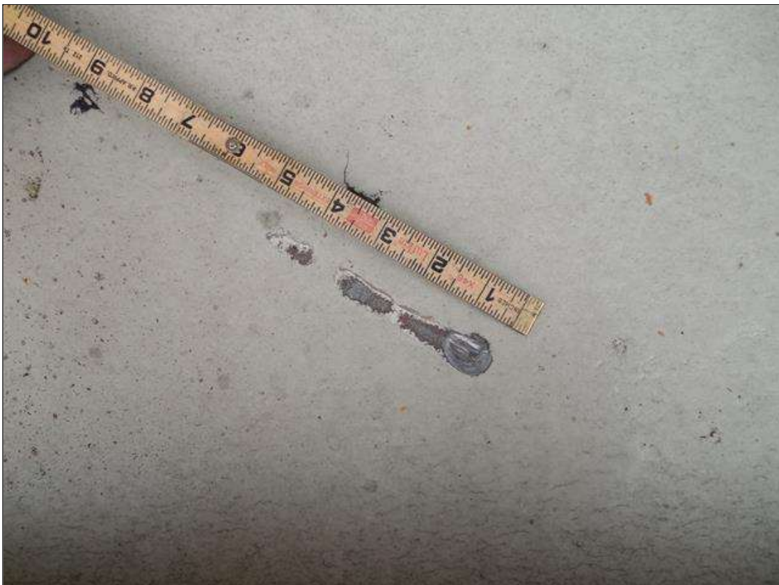
Span 4 Beam 3: APPROX 4"L x 1/2"W SCRAPE ON SOUTH FACE OF WEB, LOCATED 4-1/2" UP FROM BOTTOM FLANGE AND 19' FROM BENT 4 BEARING
